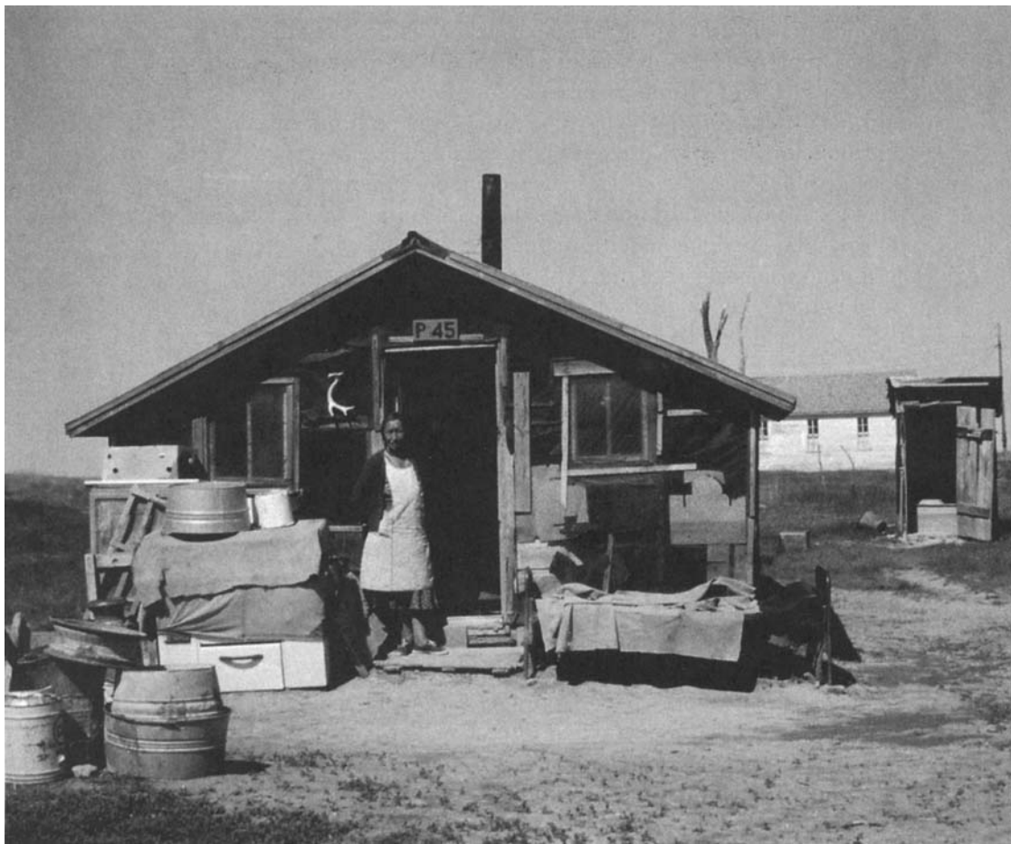
Housing conditions on the Rosebud Sioux Reservation, South Dakota, in 1970. Similar conditions prevailed at the nearby Pine Ridge reservation.
